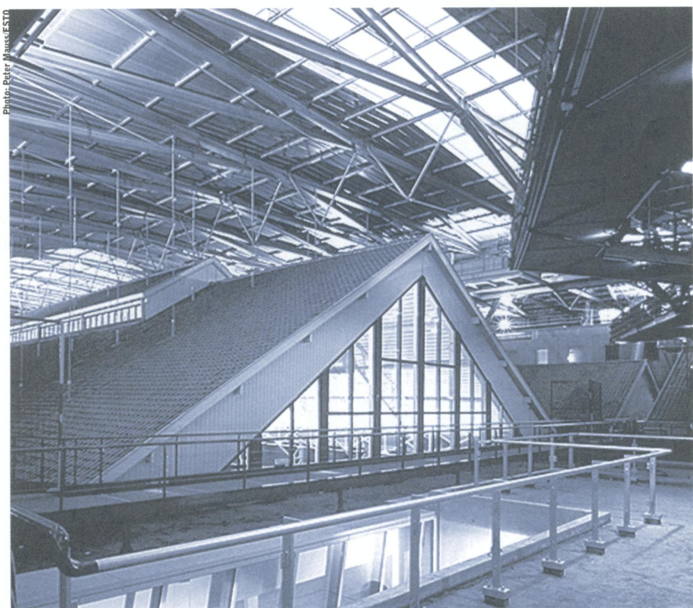
Renovated existing structure, roof overhead.
